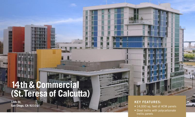
Located next to Petco Park, St. Teresa of Calcutta Villa is the largest affordable housing unit in San Diego County. The project skin consists of 14,000 square feet of blue ACM panels. To accommodate the light ACM panels with San Diego's notorious offshore winds, extensive framing was installed to ensure panels stay properly attached to the wall.
